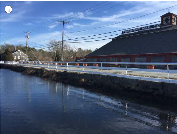
PARKERS MILL DAM, CURRENTLY CLOSED TO VEHICULAR USE
