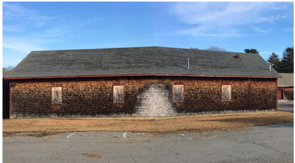
EXTERIOR VIEW OF PACKAGING BUILDING
