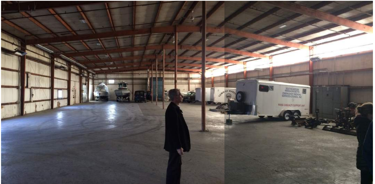
INTERIOR VIEW OF STEEL BUILDING SHOWING CURRENT USE AS TOWN STORAGE
