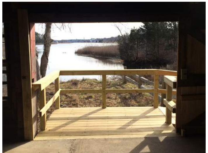
VIEW FROM MAIN SPACE TOWARDS MERCHANT'S WAY
