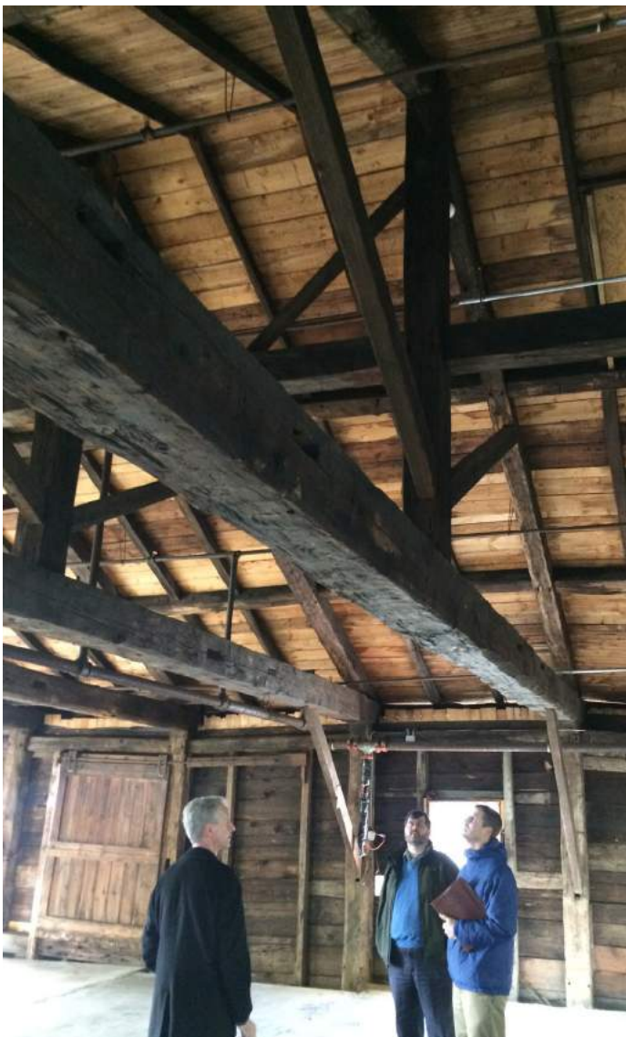
INTERIOR VIEW OF MAIN SPACE IN FREIGHT BUILDING
