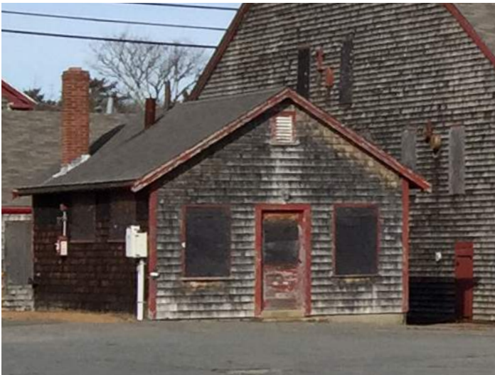
EXTERIOR VIEW OF RESTROOM BUILDING
