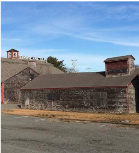
EXTERIOR VIEW OF PICKLING BUILDING
