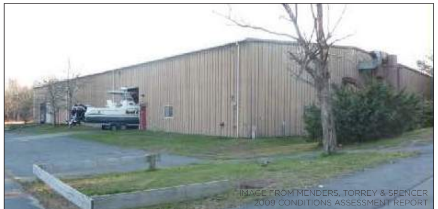
EXTERIOR VIEW OF STEEL BUILDING SHOWING ITS UTILITARIAN CHARACTER
