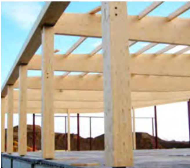
Example of a timber structure comprised of glue-laminated columns & beams
