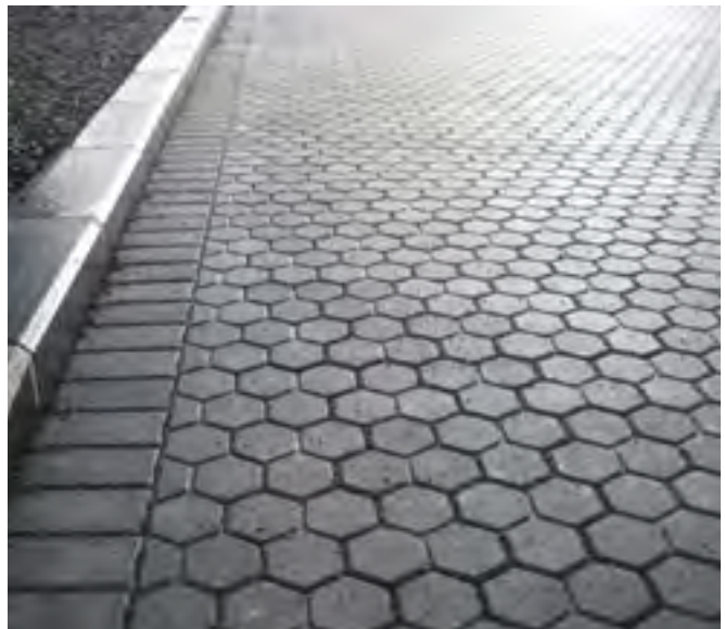
Example of permeable pavers, which can be ordered in a variety of sizes and shapes
