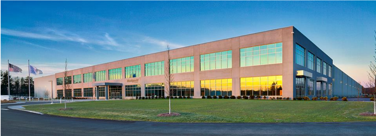
Martignetti Headquarters completed in 2017
