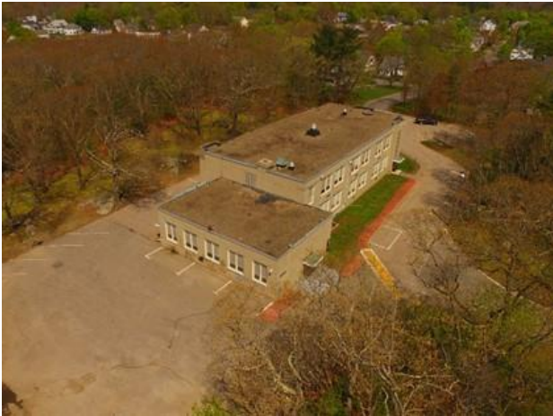
6. Overall view from the south end of the site.
