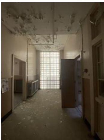
23. Second floor stairwell with glass block.
