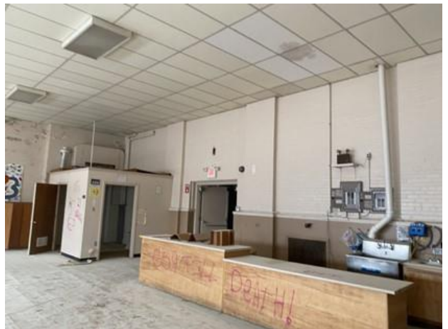
18. Existing cafetorium space.
