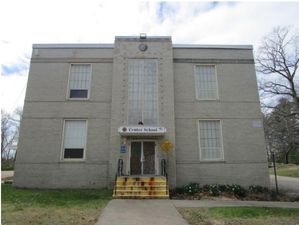
1. North elevation – front entrance.
