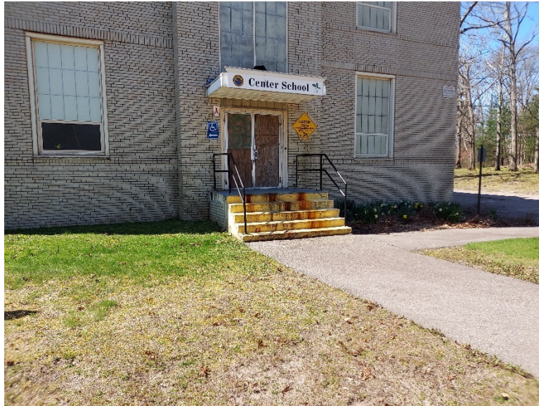
Existing Main Entry w/ Stairs
