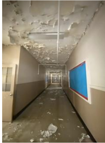
20. View of main corridor between classrooms.
