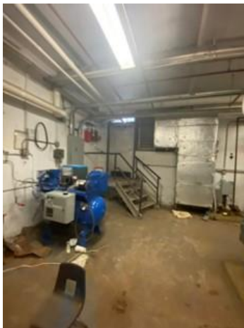
27. Boiler room exterior access to areaway.
