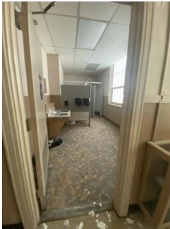
25. Existing toilet rooms.
