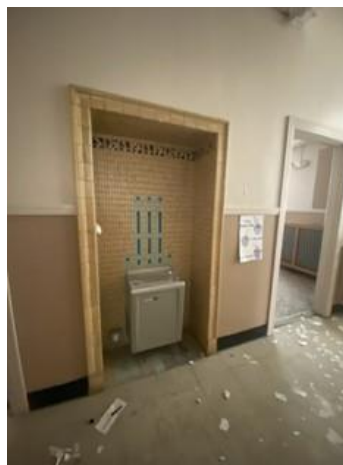
24. Tile work around water fountain.
