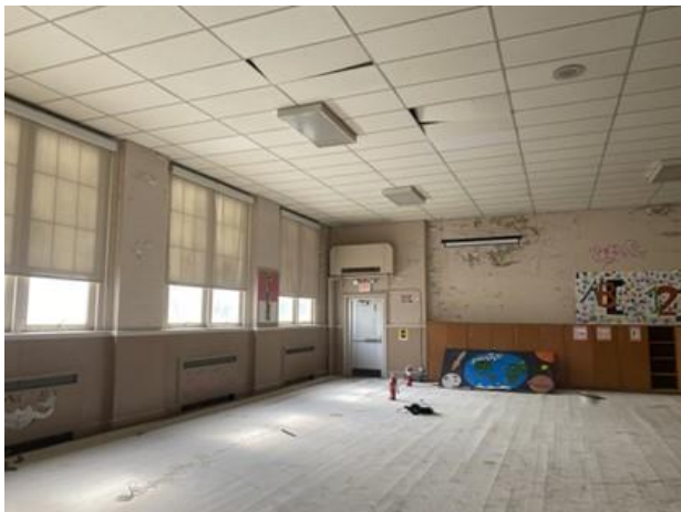
17. Existing cafetorium space.
