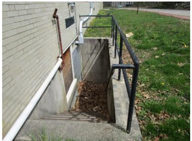
12. Areaway with stairs to basement boiler room.
