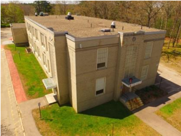
5. Overall view from northeast corner of the site.
