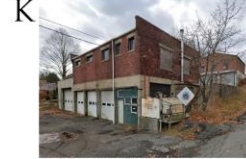
EXISTING SITE - INDUSTRIAL
