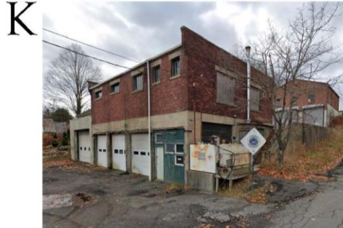
EXISTING SITE - INDUSTRIAL
