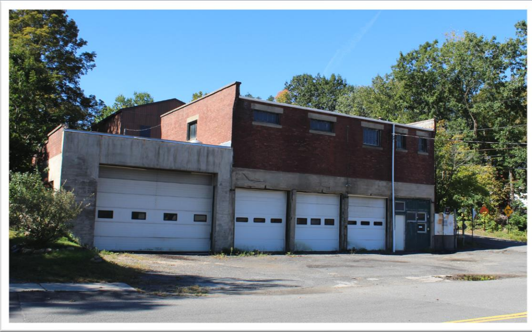
Former Buckland Highway Garage at 50 Conway Street.
