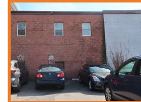
Howard Street ROW Not built Area of focus: 0.026 AC Owner: City of Taunton
