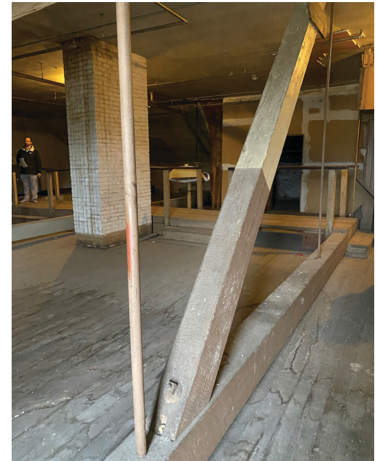
Figure 3.13. Roof trusses in the attic level
