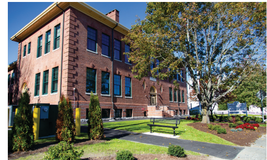
Figure 4.3. Renovation of former school building, Walker School, Taunton, MA
