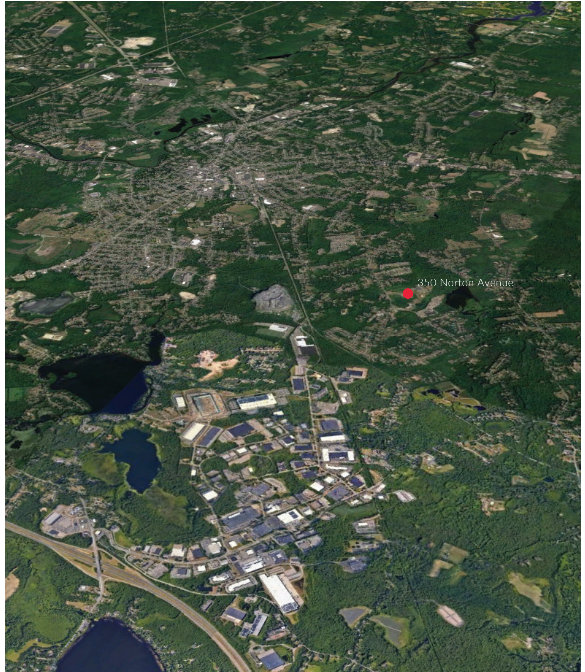
Figure 3.1. 350 Norton Avenue lies close to downtown Taunton and the Myles Standish Industrial Park (looking south).
