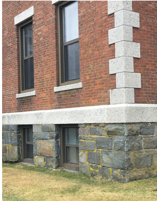
Figure 3.12. Granite details on historic building
