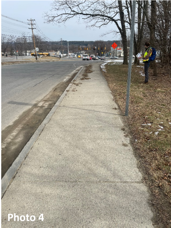
This photo is taken looking east along Wanoosnoc Road as it approaches Water Street. The sidewalk meets minimum dimensional requirements and is in good condition. As pedestrians get closer to the intersection, they turn off the sidewalk and walk along the grassy open space to the bus stop.
