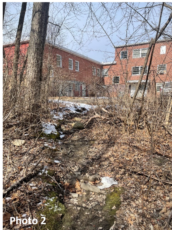
Photo 1 shows the driveway to the rear of the site with broken pavement and erosion from stormwater runoff. Photo 2 shows the back of the school building where channelized stormwater drains into the stream.
