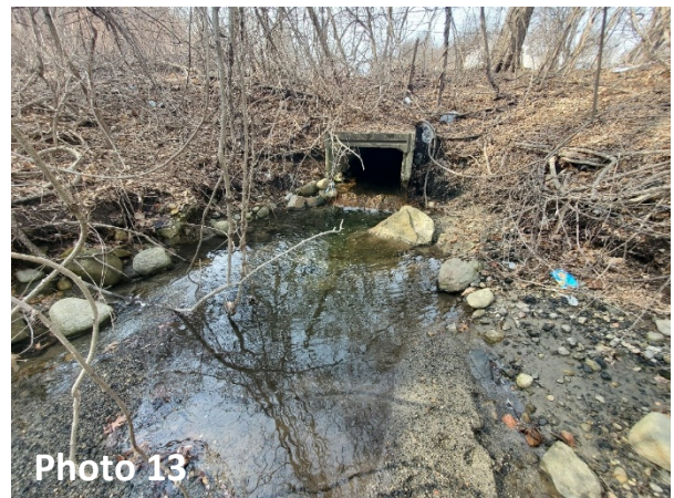
Photo 12 shows the stream leaving the site. The Water Street bus stop is visible in the background. Photo 13 shows water entering the site from Wanoosnoc Road. The deep pool in front of the culvert suggests water flow can be high volume.
