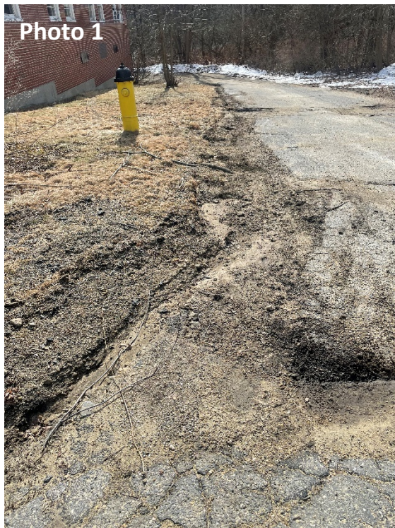
Photo 1 shows the driveway to the rear of the site with broken pavement and erosion from stormwater runoff. Photo 2 shows the back of the school building where channelized stormwater drains into the stream.
