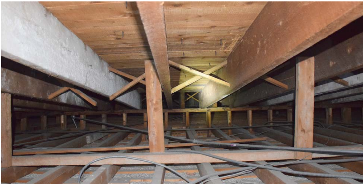
Figure 3-Roof Framing at Interior Bearing Wall
