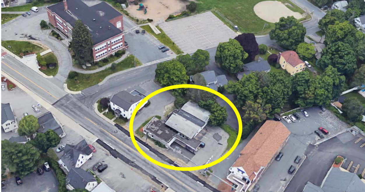
Figure 20. Aerial and street levels views of 15 Maple Avenue.
